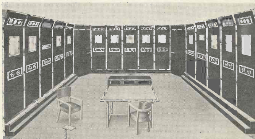
The 30-kilowatt transmitter for the new Eiffel Tower station.
